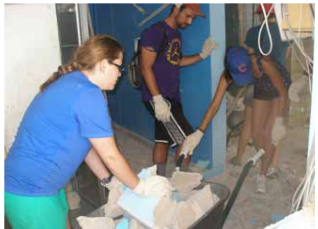
Volunteers helping with the reconstruction.
